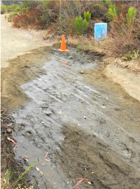
Leaking near blue fixture
