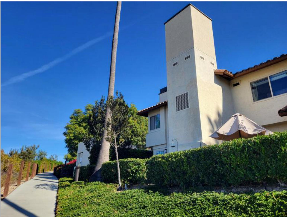
View of Antenna Structure.
