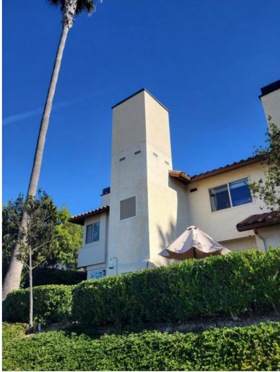
View of Antenna Structure.
