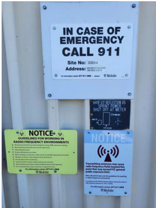
Access to Shelter Area.
