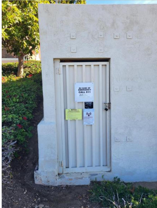
Access to Shelter Area.
