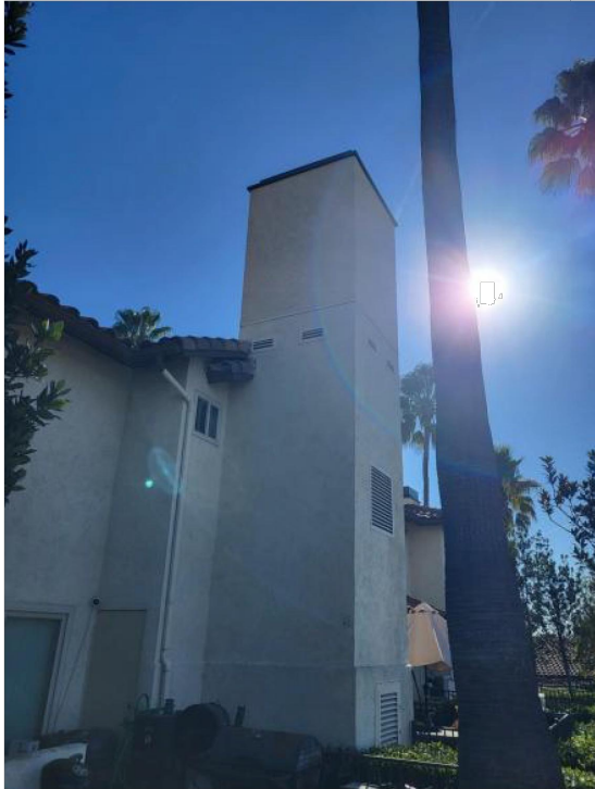
View of Antenna Structure.
